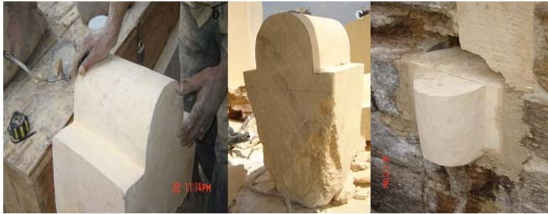
Fig. 15. Missing parts completion: a, b - Reproduction of lost Cantilever (Corbel) below the Sebil window from dolomitic limestone, c - using the reproduction corbel for façade conservation.
