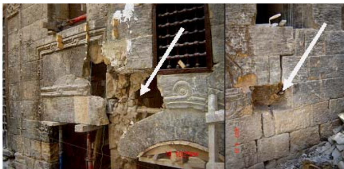
Fig. 13. Removing of all deteriorated and deformed mortar and stone blocks
