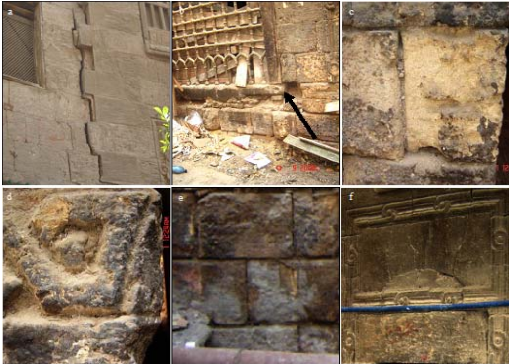
Fig. 6. Photograph of decay features common at Sebil facade a - buckling and leaning, b - deformation, brittle failure with loss of stiffness in the structure elements of the façade (lost cantilever (Corbel), c - Scars of flaking, d - hard crust and scars of flaking e -Efflorescence's to light-colored crust tracing the surface, f - soiling by particles from the pollution.
