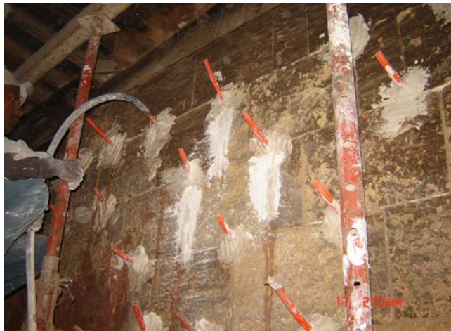
Fig. 14. Grout mixture was injected by air pressure into the open joints in the stonework at the Sebil façade and large areas of walling was need these treatment.
