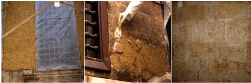
Fig. 18. Salt extraction by Sepollite poultice: a - The poultices completely covered the stone surface to a uniform thickness of about 1.0cm, b - removing the poultice, c - after restoration.
