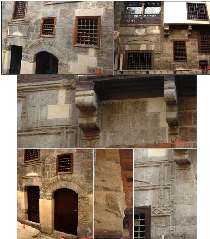
Fig. 20. The façade of the Shahin Agha Sebil and its artistic and architectural elements after restoration process.
