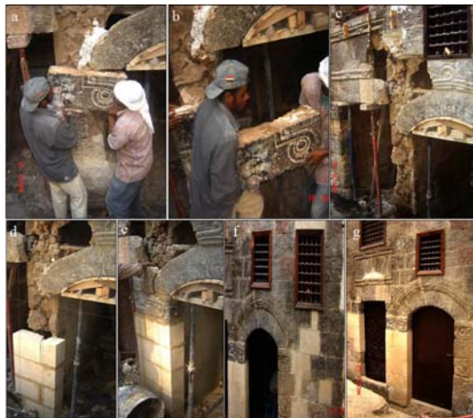
Fig. 16. Replacement and reconstructing the missing stone blocks of the Sebil façade by dolomitic limestone and lime mortar, a, b, and c - show the separation of the architectural elements paving to resistance the Multiple-leaf walls behind it, d, e - completion and replacement of the lost and deteriorated of the stone blocks at the Sebil façade, f and g - after restoration.
