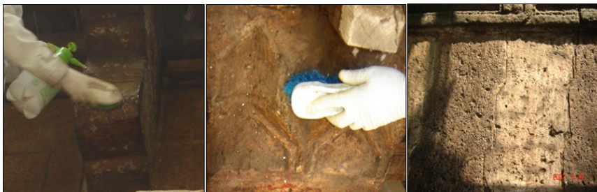
Fig. 17. Wet cleaning with warm water and soft brushes
