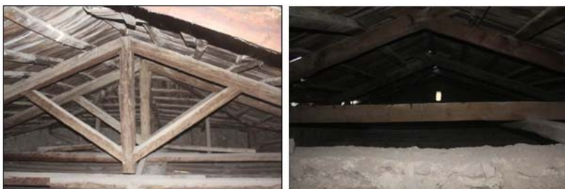
Fig. 6. The truss: a – central roof 1, b – wing roof
