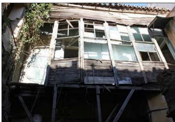
Fig. 7. Typical galleries looking in the internal open space with temporary prop
