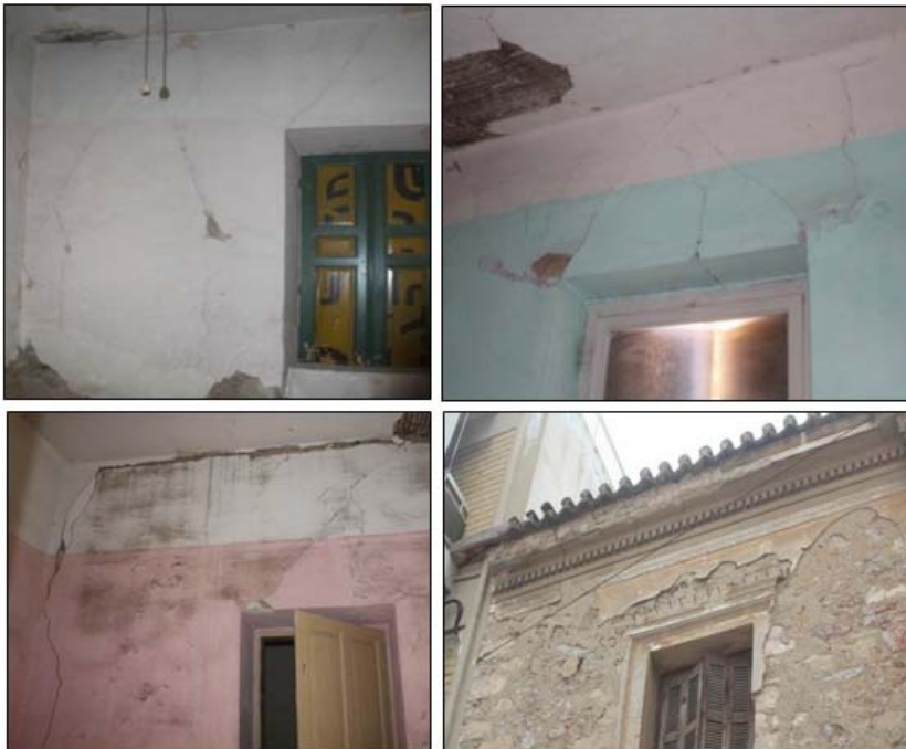
Fig. 8. Typical damage of main bearing walls from left to right and top to bottom – Cracking of wall 3 (ground floor); Lintel cracking of wall 1 (1st floor); Vertical crack of wall 6 near wall connection (1st floor); Cracking of wall 2 at top of building
