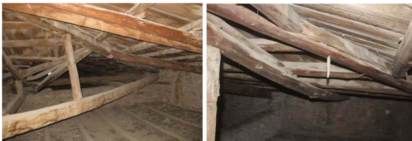
Fig. 10. Excessive truss deflection and typical failure of truss member
