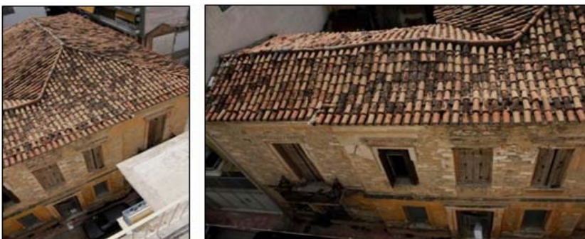
Fig. 5. Building's roof: a – central roof 1, b – wing roof
