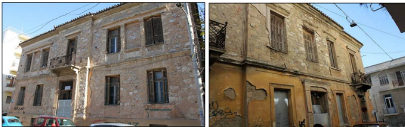
Fig. 4. Building façade: a - wall 1, b – wall 2 (Northern face)
