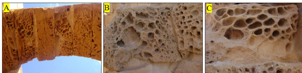
Fig. 2. Honeycomb weathering at the Leptis Magna: A and B - honeycomb weathering developed along inclined bedding in limestone; C - honeycomb weathering in homogenous limestone
