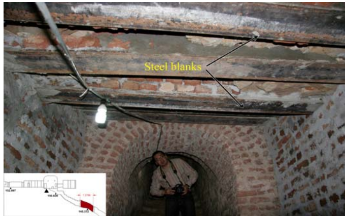
Fig. 7. Supports at the first few meters of the tunnel
