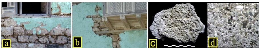
**Fig. 21.** External collapsed wall plaster of green color (a and b), The texture of the Qasr El-Emara wall plaster (c and d).
