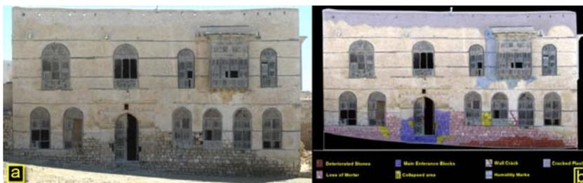
Fig. 6. Main façade of the Qasr El-Emara building (a) and its deterioration map (b).
