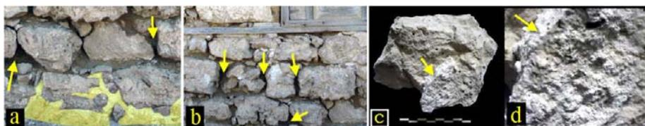
Fig. 19. Lack of mortar between stones (a and b), adhered mortar to the building stone (c and d).
