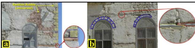
Fig. 5. Random rubble "un-coursed" method (a) and windows openings with rendered cut-stone arches (semicircular) (b)
