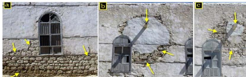
Fig. 7. Loss of wall plaster layer from ground level up to 2 m high (a) and deterioration of the wall plaster layer (b,c)
