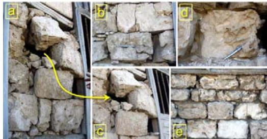
Fig. 10. Partial collapses and penetrative cracks
