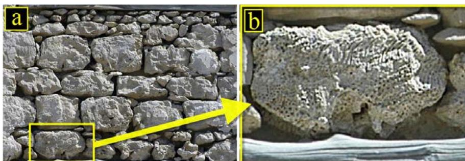
**Fig. 12.** Honeycomb coral limestone in the wall (a), detail of a coarse texture honeycomb coral limestone (b)
