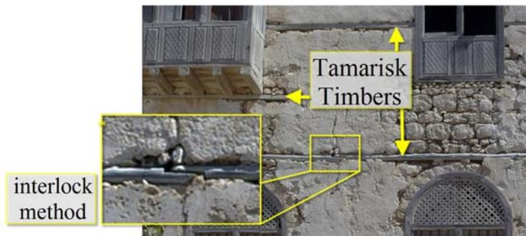
**Fig. 26.** Horizontal timber that supported the rendered coral wall and the half/half interlock method used to connect timbers
