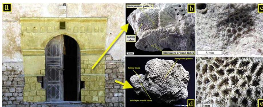
**Fig. 11.** Main façade having two kinds of honeycomb coral limestone (a), fine texture honeycomb coral limestone (b and c), coarse texture honeycomb coral limestone (d and e)
