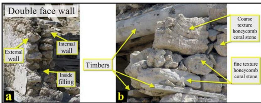
Fig. 3. The double face wall technique (a) and some of the Qasr El-Emara building materials (b)
