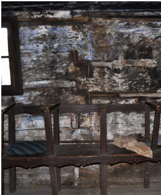
Fig. 3. Old joint, from where was enlarged the North wall of narthex
