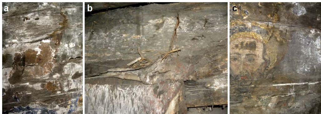
Fig. 7. Degradation of paintings layers and interstitial canvases: a - Narthex, b - nave, c - altar
