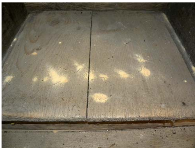
Fig. 6. – Anobium punctatum attack on boards' floor
