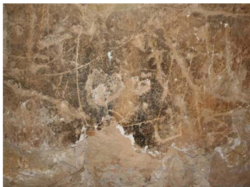
Fig. 5. The effects of salt crystals on both painting and mortars
