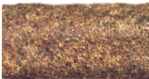
Fig. 32. External layer of the corrosion crust.
