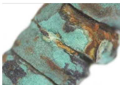
Fig. 26. External layer of the corrosion crust formed on coils, 40X.
