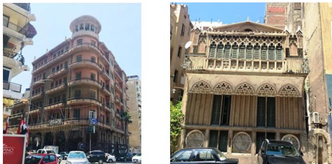
Fig. 5. The Kolovic Building (a) and De Lesseps's Villa (b)
