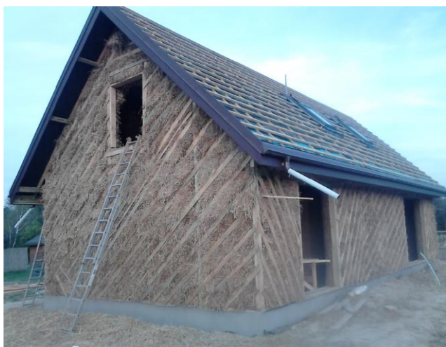
Fig. 1. Photo of a straw bale house during construction (Lublin area, Poland, 2017)
