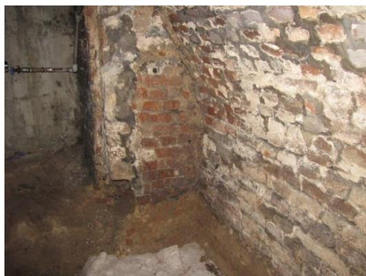
**Fig. 5.** Dampness and biological corrosion – moulds
