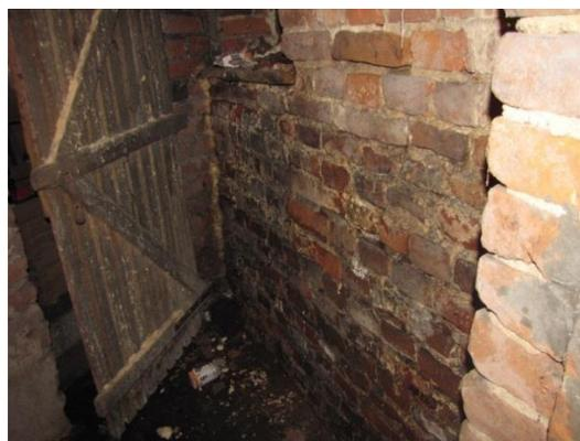
**Fig. 6.** Visible dampness and loss of joints and bricks, crystallisation of building salts
