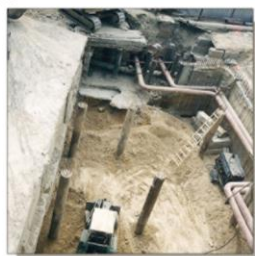
d. The process of strengthening the foundations.
