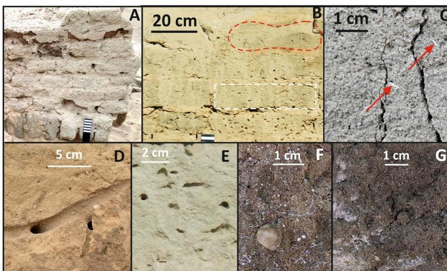
**Fig. 6.** Manifestations of mud brick deterioration (see text for details): A – exfoliation, B – deformation visible in the wall of Mustafa’s House (white dashed line indicates non-deformed brick, red dashed line indicates deformed brick), C – salt crystallization (arrowed), D – borings, E – borings, F – salt crystallization (white threads and points), G – saline efflorescence on the surface.
