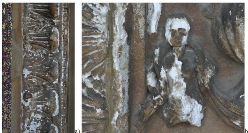
**Fig. 2.** Particular of piers: a) state of conservation of the marble with salts efflorescence, sugaring, powdering, black crust, browning of the surface due to the previous covering; b) losing of the flourishing shape due to the effect of the salts efflorescence with following sugaring and powdering of the marble.
