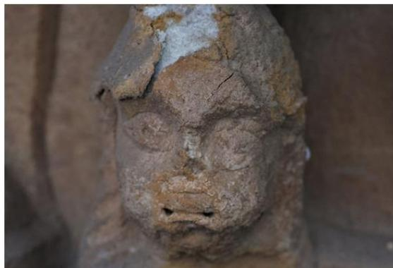
**Fig. 3.** Particular of a capital. Losing of the carving due to the action of the ageing of a synthetic adhesive applied in a previous restoration.
