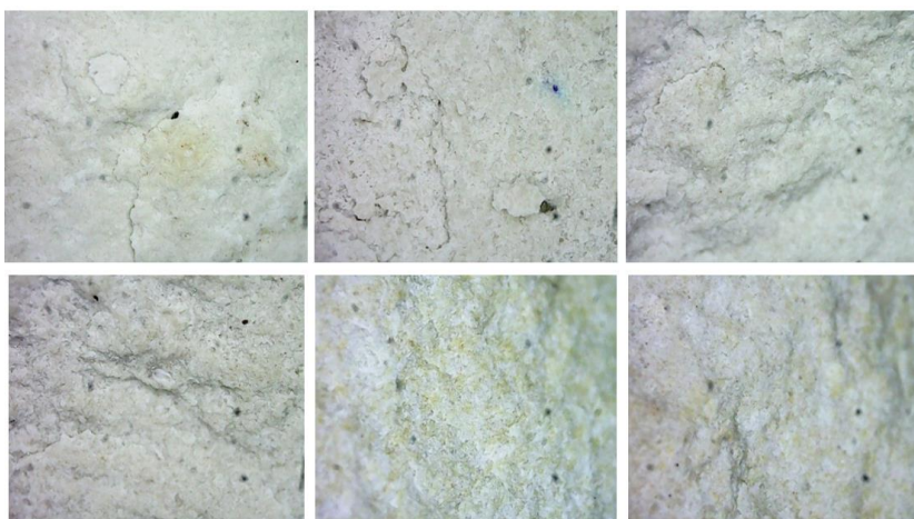
Fig. 3. The visual study with light microscope of samples of stone walls. The samples showed cracks and decomposition of the surface and sample of the pillar
