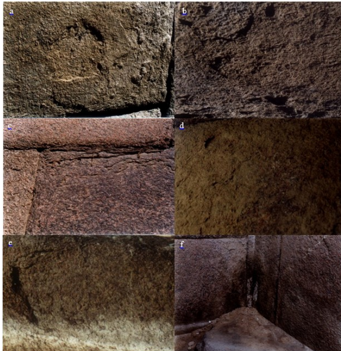
Fig. 1. Extensive deterioration features of granitic casing of Valley Temple;
