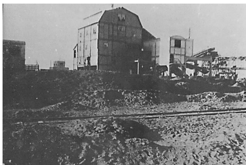
Fig. 2. View on the colliery of Kenadsa
