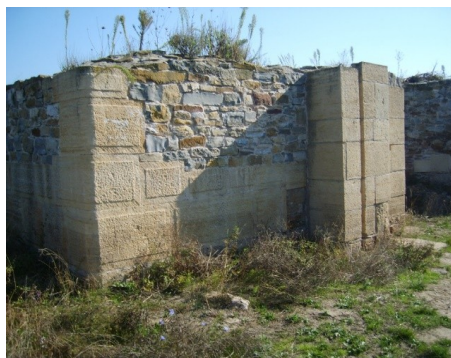
Fig. 2. Consolidation-restoration of the fortress walls.
