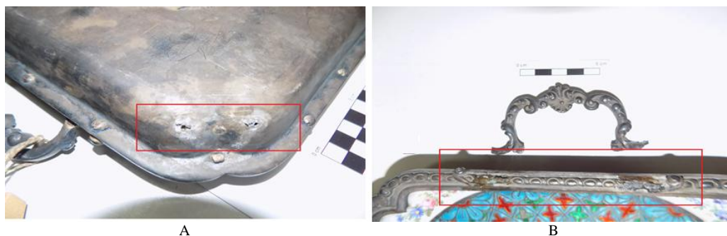
Fig. 7. The areas where the solder was applied, the broken legs (A) and the broken handle (B).
