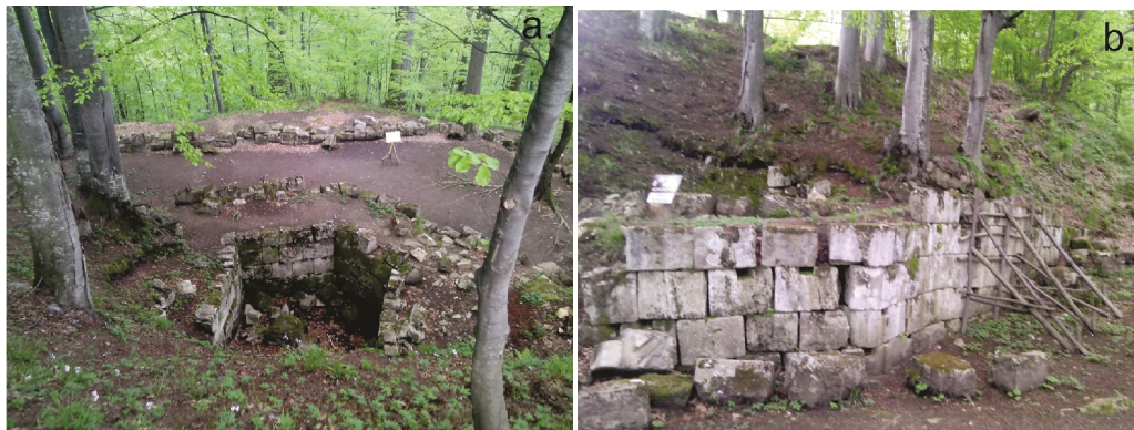
Fig. 5. Structural-functional instability and deterioration of immovable heritage: a. Root wedging affecting the walls from the eastern slope of Dacian Fortress – Sarmisegetusa (a UNESCO World Heritage Site, ID 906-001) from the Orăștie Mountains, Hunedoara County, Romania. b. Basic measures to stop the collapse of the fortress walls
