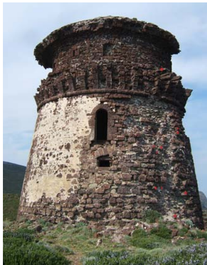
Fig. 4. In the conical base, left side of the image, remains of the covering plaster still with good adhesion of the masonry, are visible; on the right side it is evident the zone where a portion of the external wall fell, uncovering the wall core structure. With red asterisks are marked the stone blocks that in 2010 were still on site and that in the 2013 survey fell down.
