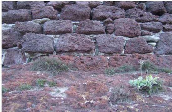
Fig. 3. The masonry made of volcanic rock blocks roughly shaped and put in place with an abundant mortar, made necessary by the irregularities of the same blocks
