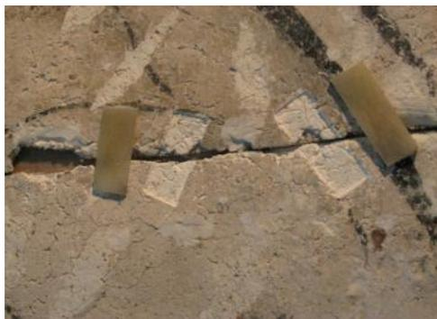
**Fig. 15.** Assembly system of the two sections of the back panel.
