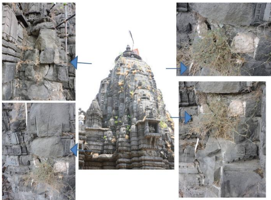
Fig. 1. Photograph showing the effect of vegetation on the Sundarnarayan temple, Nashik
