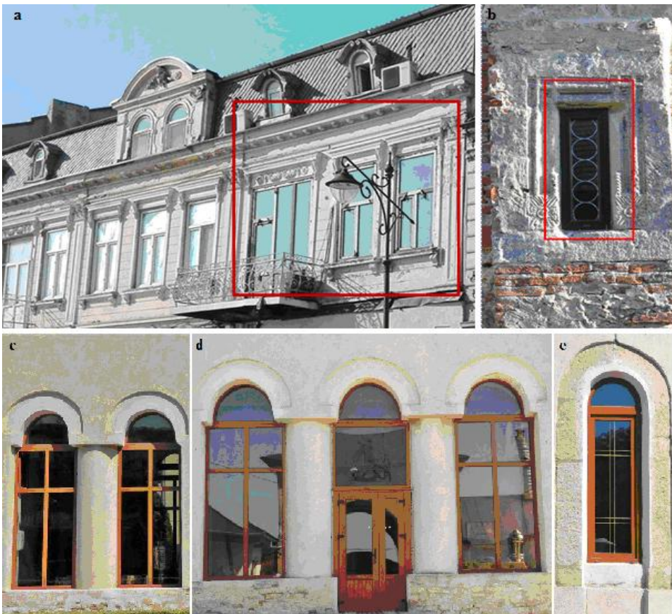
Fig. 2. Rehabilitation/modernization using thermo-insulated glass: a – Building on Tomis Boulevard, Constanta, Romania (personal photo, July 2016); b – Hadâmbu Monastery church, Schitu Hadâmbului village, Mireneasa commune, Iasi County, Romania (personal photo, July 2016); c, d and e –Hlincea Monastery church, Iasi county, Romania (personal photo, august 2016)
