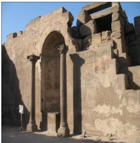
Fig. 3. Interior view of the church at the Luxor Temple
