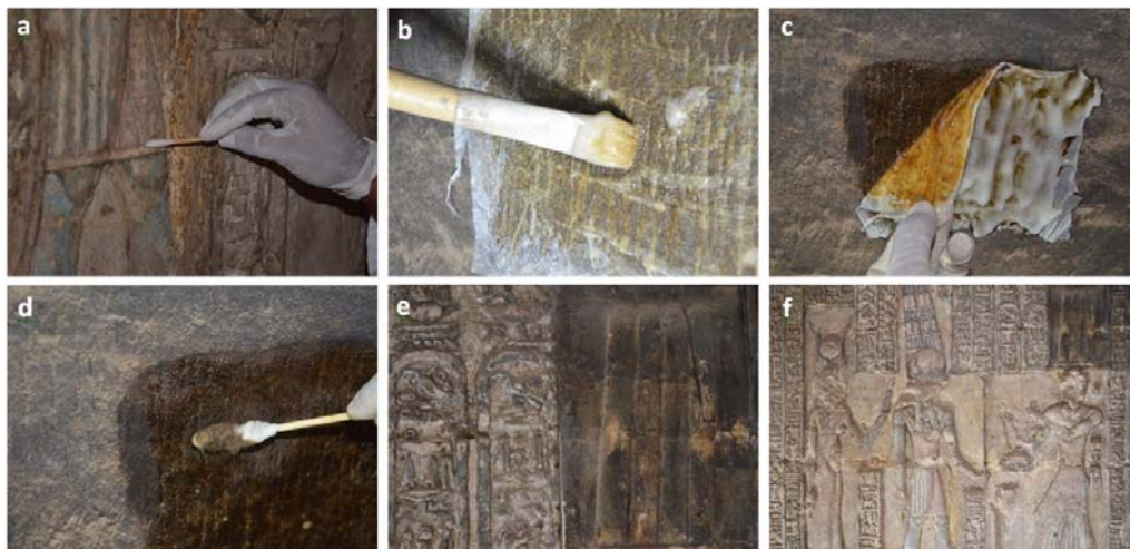
Fig. 14. Application of ZnO NPs on mural painting in the temple of Isis: a -cleaning by ZnO NPs with soaked in a swab; b - The wet pulp is manually distributed over the Japanese paper layer; c - Composite (3); d - removing of poultice; e - removing of remaining materials with cotton swab embedded with distilled water; f - the results of mechanical and chemical cleaning.
