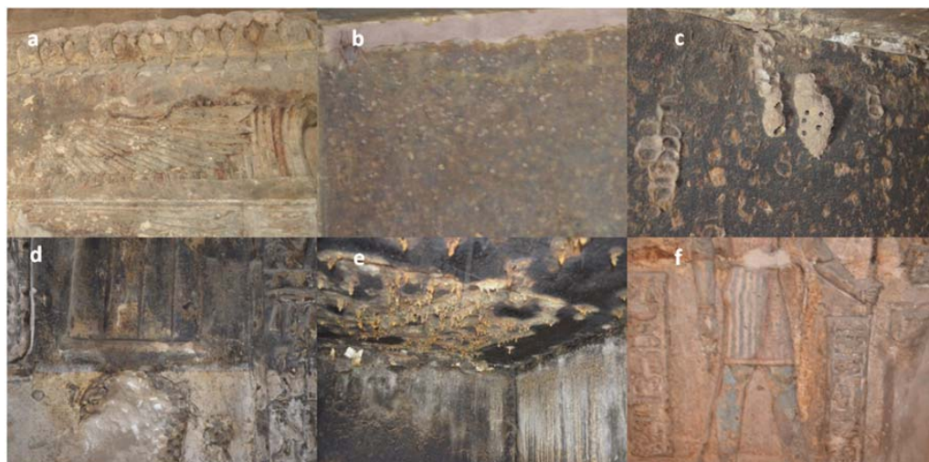
Fig. 2. Conservation state of the Isis Monastery, showing the high degree of decay of the sandstone: discoloration of the surface, bats dropping, concentrated layer from dust, wax and birds, bee nests, spider web nests, soot, oil soot layer and losses of pigments.
