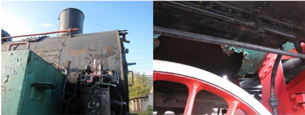
Fig. 6. Surface corrosion (left) and structural corrosion (right) on a locomotive at the Warsaw Railway Museum.
