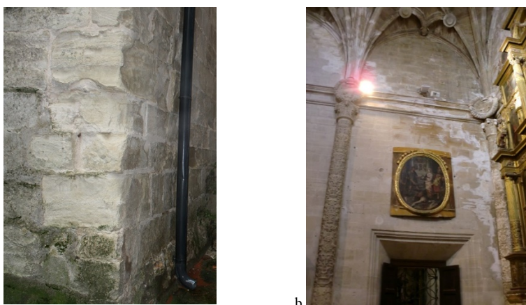
Fig. 2. Common pathologies in the Stone of Arcos de la Cantera located at the Cathedral of Cuenca: a - Alveolar erosion, b - Salt efflorescence
