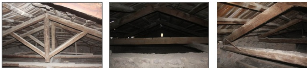
Fig. 6. Truss of central (left and right) and wing (middle) parts of the roof
