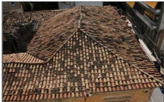
Fig. 5. Roof of Aktaiou building
