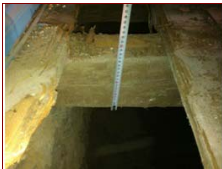
Fig. 4. Floor wooden beams
