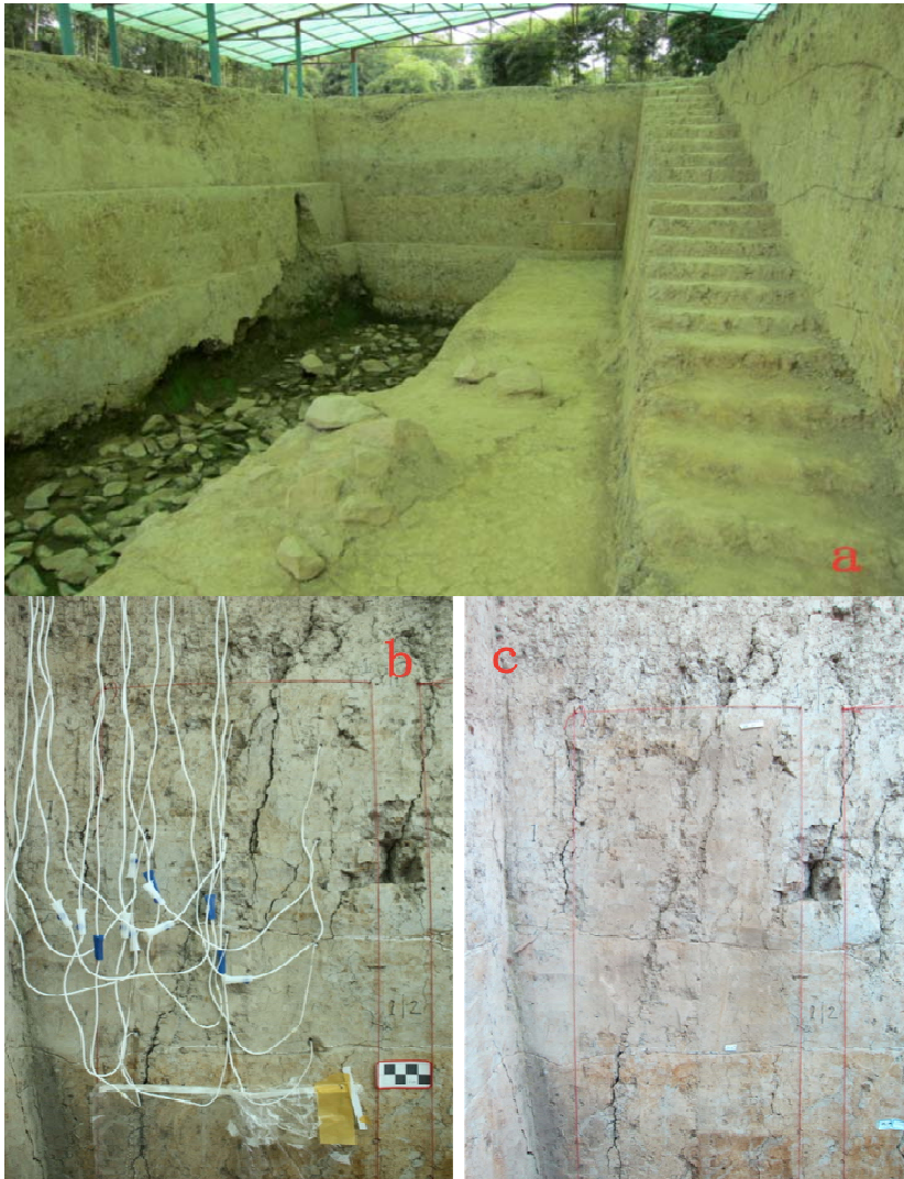
Fig. 5. Pictures of ancient Liangzhu city wall consolidation work: a - north city wall relic of Liangzhu, where the consolidation work was performed; b - Injecting the consolidant using perfusion tubes; c - the consolidation area one month after the treatment.
