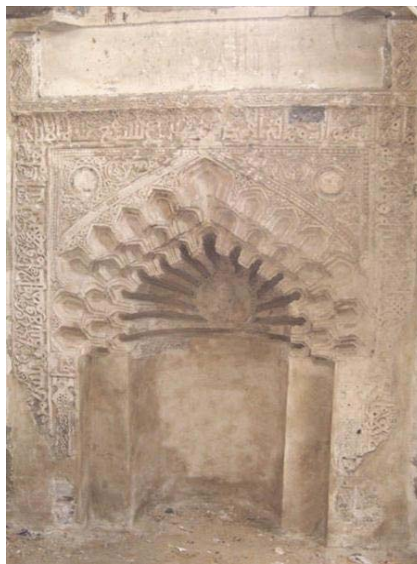
Fig. 12. Al-Hasawati stucco mihrāb after the consolidation
