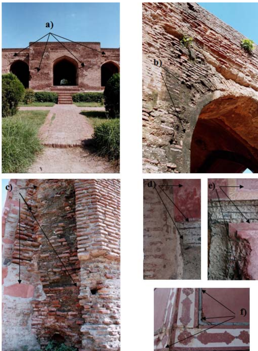
Fig. 1. Deteriorated façades of Nur Jahan Tomb: a) Rear façade with cracks, b) Biological growths, c) Jointing locations of historic and repair masonry, d) Lime-Cement mortar interface, e) Cracks in repair masonry and f) Cracking and rusting of repair works with cement mortar.
