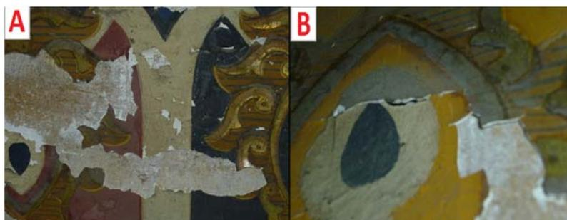
**Fig. 1.** Deteriorated wall paintings: various deterioration phenomena which can be seen within the painted layers in the chamber wall of Khediew Tawfik's mother Nour Shafaq in Hawsh al- Basha building.
