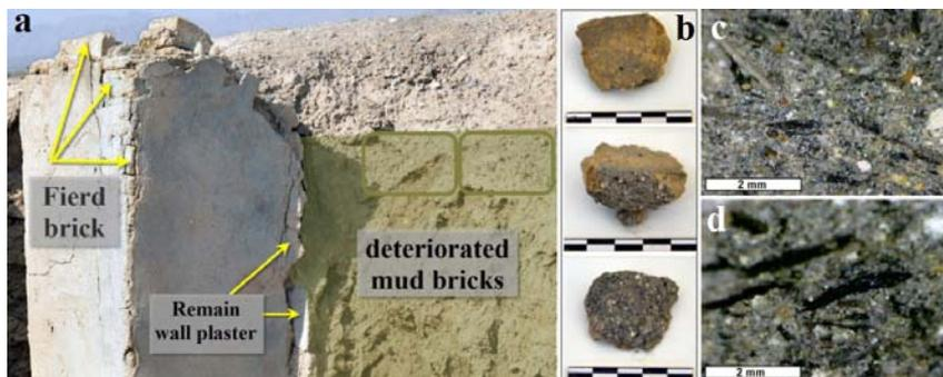
Fig. 11. The stable plaster layer on the burnt pillar, and the remains of plaster on the mud brick wall (a) and the composition of the sample MP.10 (b, c, d)
